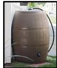
If your rain barrel is covered (and it should be), it will also need an opening through which excess water can escape.
